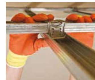
Sto primary & secondary channels installed.
