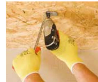
Sto strip hangers fixed to substrate using suitable fixings.
