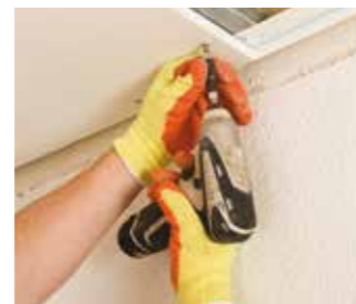
StoSilent Distance boards fixed to SC400 grid & AP profiles using suitable dry wall screws.
