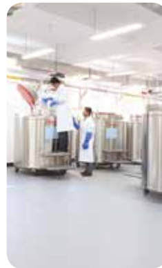
Chemical Storage Areas
