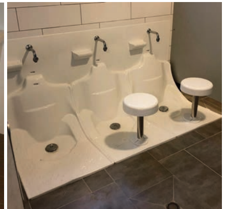
WM MODULAR SHOWING A DISABLED UNIT FOR WHEELCHAIR ACCESS
