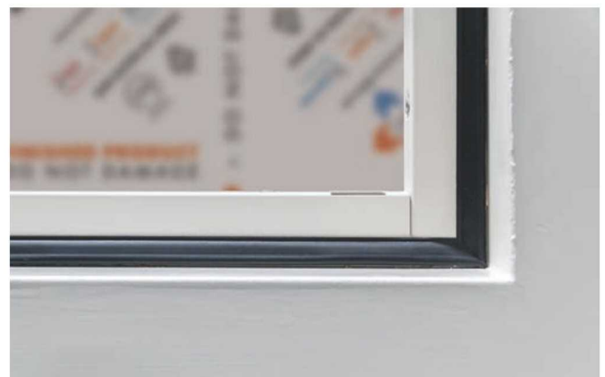
Intumescent smoke seal prevents the passage of smoke and hot gases
