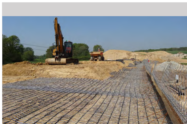
ParaDrain® used with Green Terramesh®
