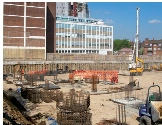
The watertight basement measures 80m x 70m x 4.5m deep
