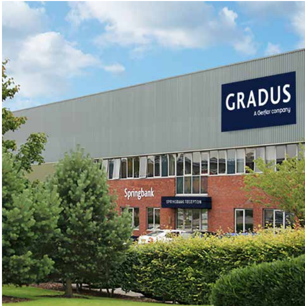
Gradus Springbank - Manufacturing plant for our Accessories products Macclesfield Cheshire UK
