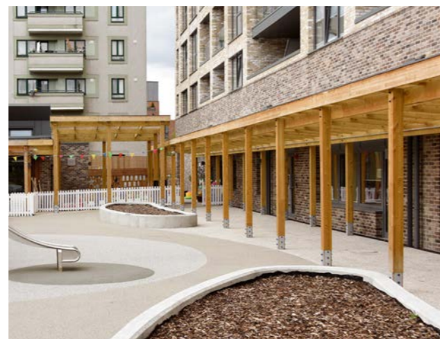
Delamere Timber Walkway BXDB/DEL/MONO-WALK
