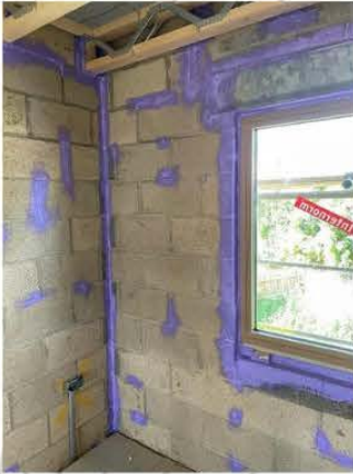
2.2.9. Internal brick connections
