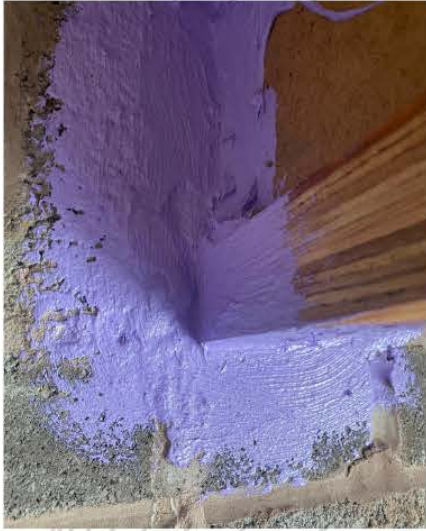
5.1.2 Joist connection into masonry wall
