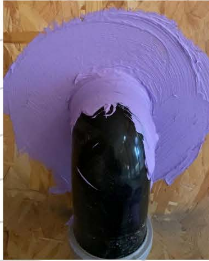
5.1.3 Pipe connection through timber frame
