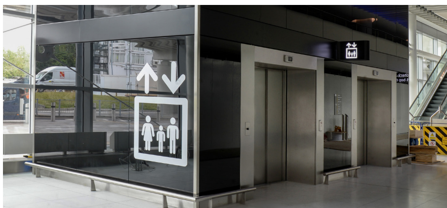
Above: Manchester Airport Terminal 2: Seamless interface between StoVentec Glass and MICAM panels
