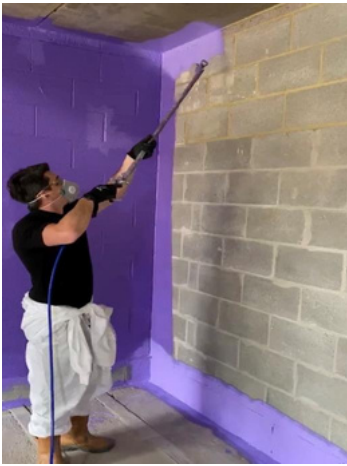
Passive Purple spray install.
