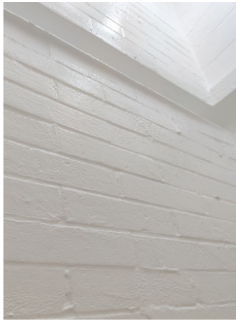
Passive Purple Airtight White Edition retrofit.
