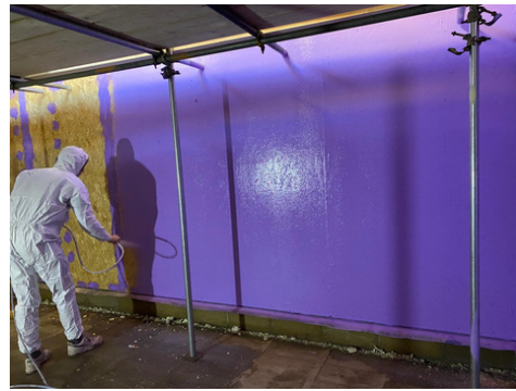
Timber frame wall.
