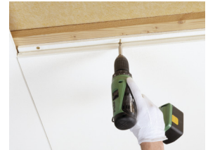
Master F is installed by screw fixing
