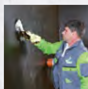
Waterproofing against Radon
