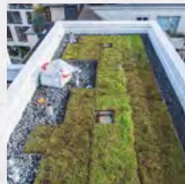
Under ballast / green roofs
