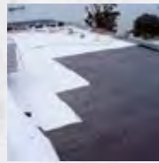
Waterproofing on bitumen
