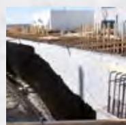
External basement waterproofing
