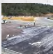
Floor slab waterproofing
