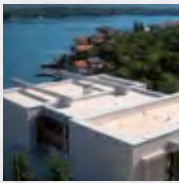
Liquid roof waterproofing
