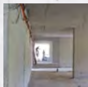
Large surface restoration
