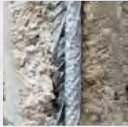
Corrosion protection (coating)
