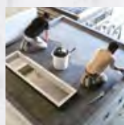
Precast concrete production
