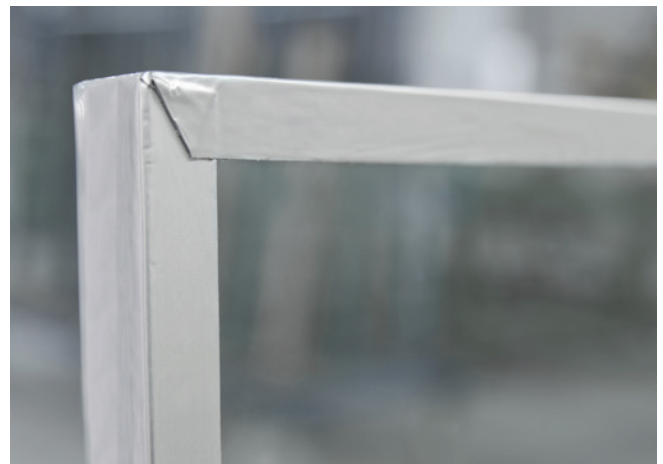
PYRANOVA® with intact edge protection sealing tape (silver)
