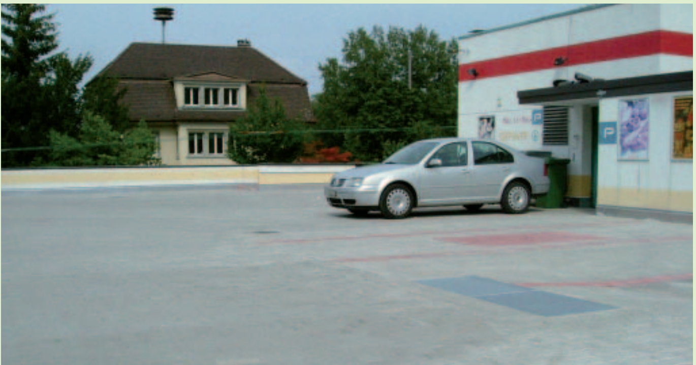
A drivable roof deck
