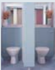
Cubicle with Half height framed duct panel system
