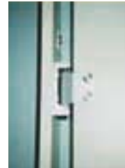
Door hinge can be fitted to close, or if required, self open. Designed to clamp and through fix. Can be set for door to be lifted off or permanently fixed. Set clear of pilaster, therefore avoiding trapped fingers
