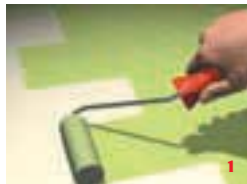
1 Paint subfloor with Primer
