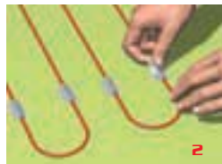
2 Lay out heating element
