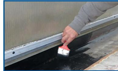
Effisus Contact Adhesive is a ready-made contact adhesive for the high-performance bonding of Effisus Ecofacade membranes to all conventional mineral construction substrates (concrete, breeze and aerated concrete, chalky sandstone, brick, clinker, plaster), PVC, aluminum or timber. Suitable for smooth and even substrates. In combination with the Effisus Coat NP Primer bonding operations can be carried out at temperatures down to -10°C and on damp (absorptive) construction substrates.
