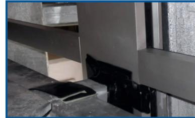
The Effisus Bond GF tape is the efficient and sustainable solution for sealing details on surfaces with irregular shapes and configurations. Effisus Bond GF is an adhesive tape, with exceptional adhesion properties. The adhesive is kept unaltered by a PE transparent film, and the tape is highly elastic and extensible (longitudinally and transversally). It has perfect adherence to Effisus VCL's, Effisus Breather membranes and Effisus Ecofacade Membrane.
