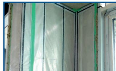
Effisus VapX Membrane is a one-ply vapour control layer (VCL) designed for facades, in order to build an airtight and vapour barrier avoiding condensation risk and improves the building airtightness.
