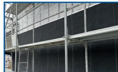
Breathable membrane made of a special polypropylene microfiber for moisture management and protection of the facade against driving rain and moisture minimizing condensation risk.
