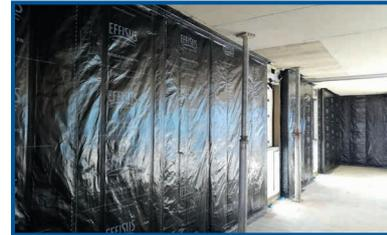
The Effisus Vapour FR is a high quality and multifunctional weatherproofing vapour barrier made of a special fiberglass technology with an aluminum foil, developed to achieve a fire reaction Class A2-s1,d0 according to EN13501-1:2007+A1:2009. The final fire classification was obtained for Effisus Vapour FR with Effisus accessories (tapes and adhesives) tested as a system.
