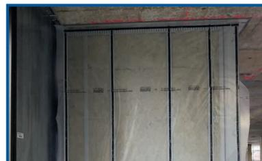
The Effisus 2Bond GO Tape is a double-sided adhesive butyl tape with excellent adhesiveness to the most common construction materials. It can be used for sealing operations between two surfaces or nail/screw penetrations, adhering perfectly to Effisus Ecofacade and Effisus VCL membranes.
