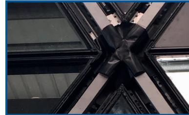
Rainscreen cladding systems sometimes are part of complex architectural facade design that implies difficult sealing that are potential leaking spots and truly challenging when it comes to ensuring a proper and efficient sealing. Great amount of costs and very time-consuming tasks are always part of addressing such challenges.
