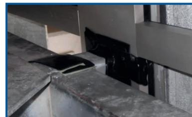
The Effisus Bond GF tape is the efficient and sustainable solution for sealing details on surfaces with irregular shapes and configurations. Effisus Bond GF is an adhesive tape, with exceptional adhesion properties. The adhesive is kept unaltered by a PE transparent film, and the tape is highly elastic and extensible (longitudinally and transversally). It has perfect adherence to Effisus VCL, Effisus Breather membranes and Effisus Ecofacade Membrane.
