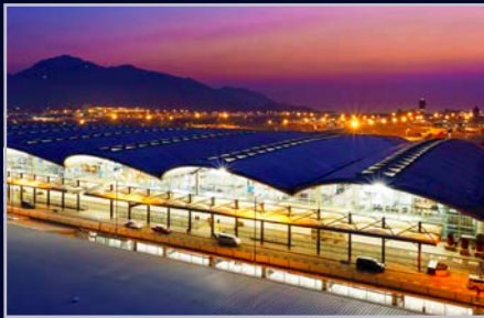
Hong Kong International Airport
