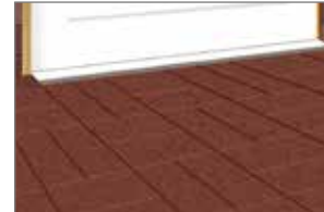
Step 4. Protective film on gratings should now be removed. Complete the installation by sealing between the door sill and grating.
