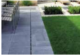
Slot Drainage
