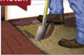
Step 1. Dig trench 100mm wide by 210mm deep for channel. Remove cap from outlet.
