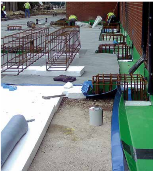
Installing Proofex Engage water proofing membrane
