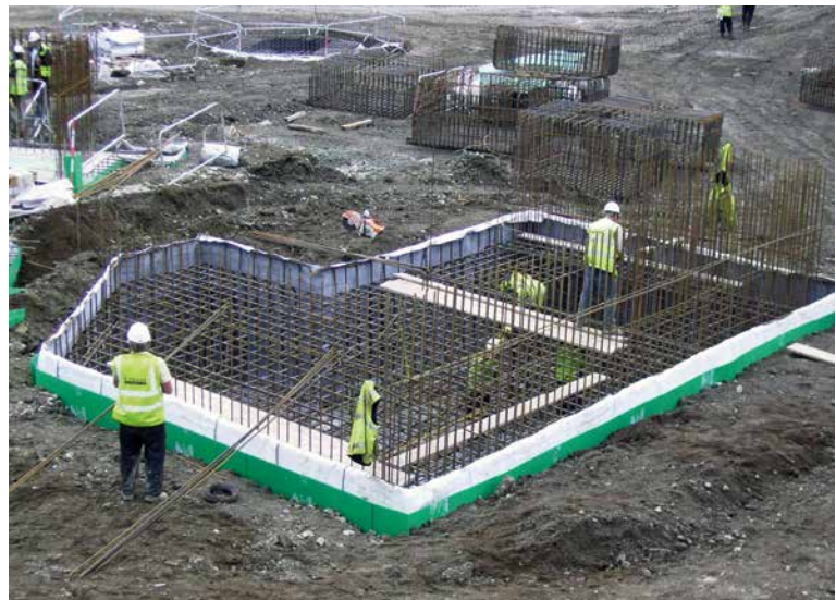
Proofex Hydromat installed inside Corriform formwork
