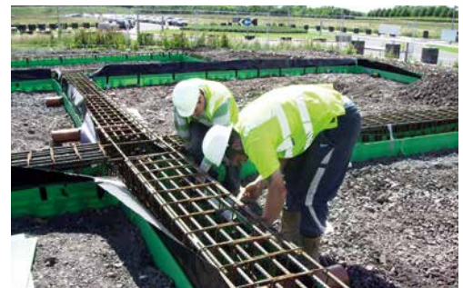
Attaching Fosroc Proofex Total gas membrane to ground beam.
