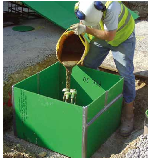
Sealing Pile Head with Supercast EPT epoxy
